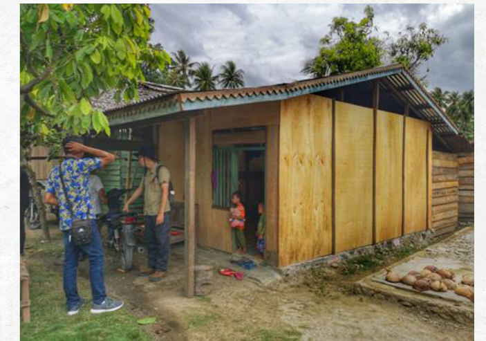
Palu. Completed transitional housing. The government will construct permanent homes adjoining these structures which can then be converted into a kitchen or storeroom.
